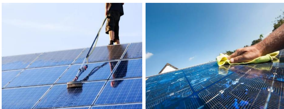
Figure 30. Illustrative Views of Panel Cleaning 40
